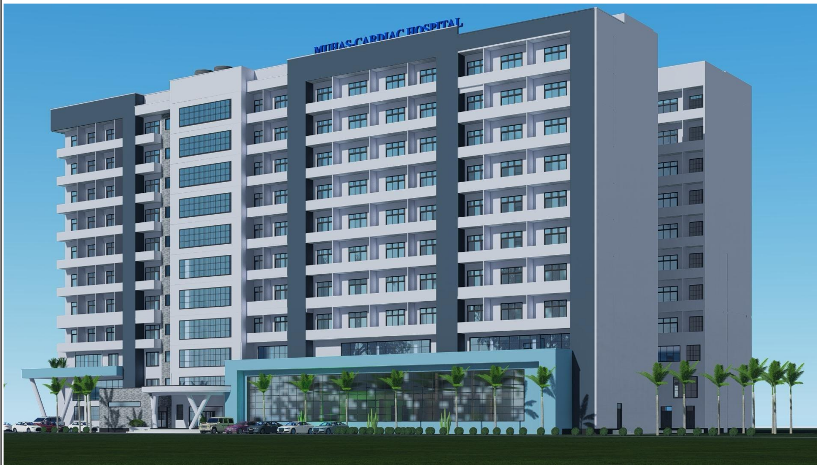
VIEW AT RIGHT SIDE ANGLE-CARDIAC HOSPITAL BUILDING
