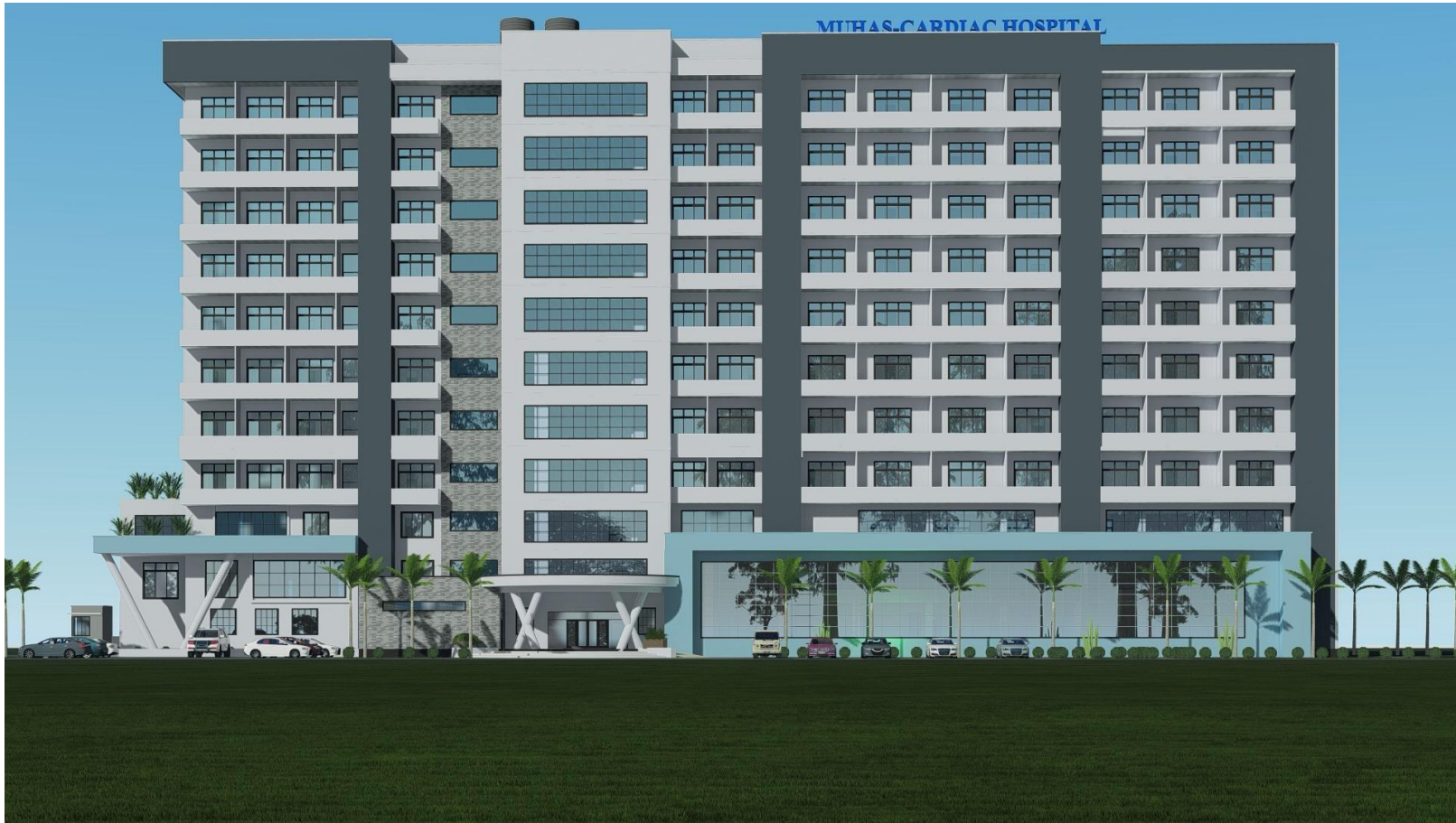
FRONT VIEW-CARDIAC HOSPITAL BUILDING
