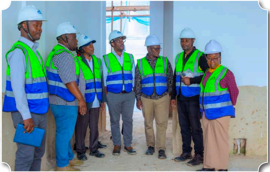
The MUHAS Audit Committee inspecting the progress of the construction progress.
