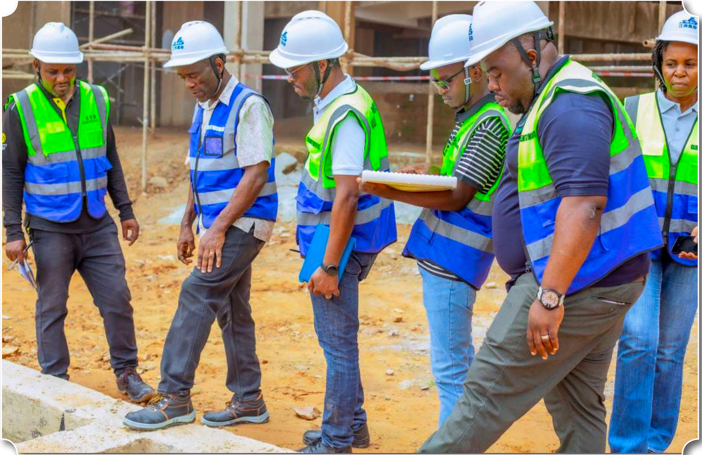
Construction inspection at the Kigoma Campus led by the Vice-Chancellor.
