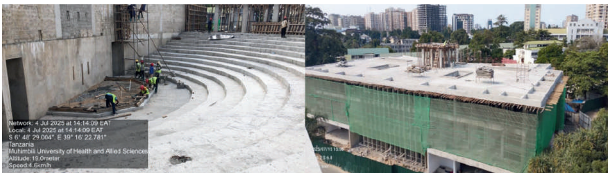
Ongoing construction of the Lecture Theatre and Office Complex at Muhimbili Campus
