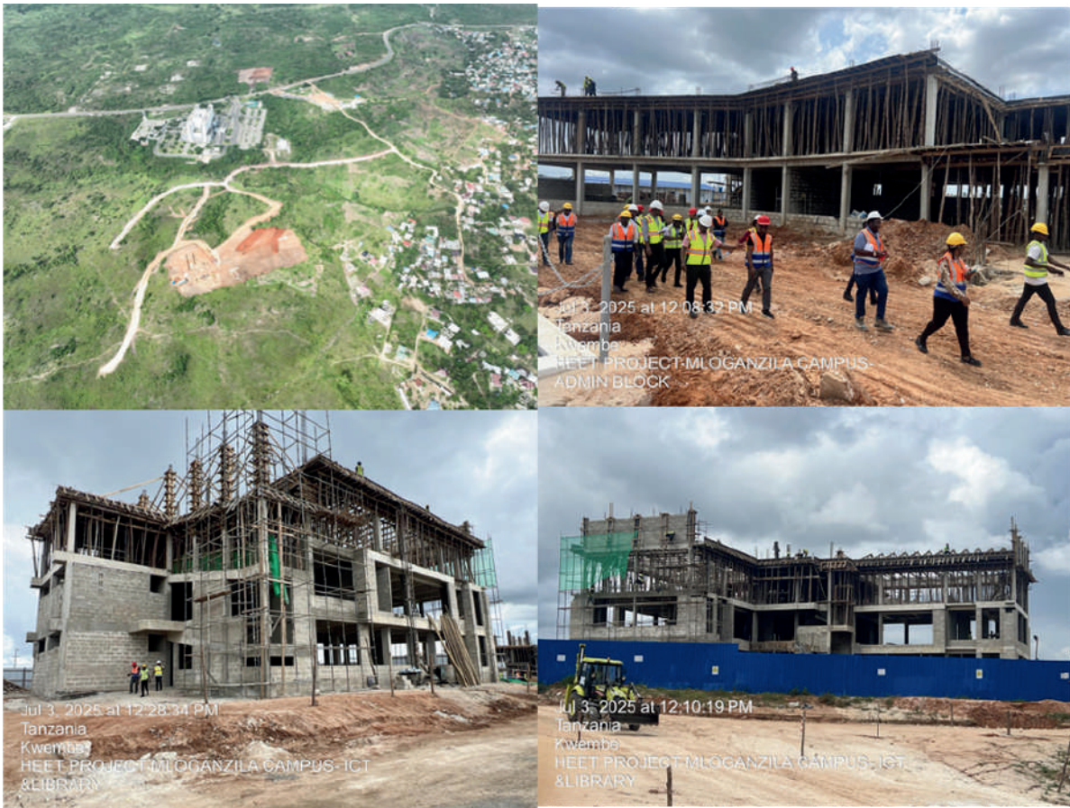
Ongoing construction of the College of Medicine at the Mloganzila campus
