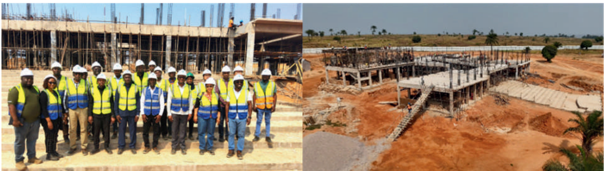
Ongoing construction at Kigoma Campus
