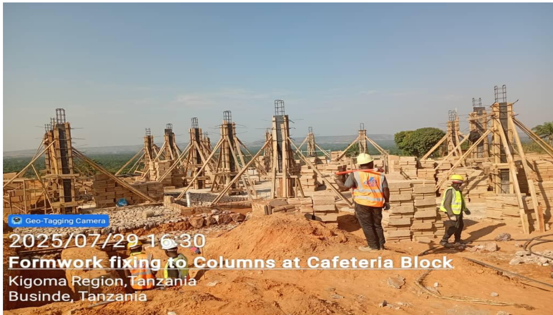
Plate 2: Formwork fixing to columns in the Cafeteria Block.
