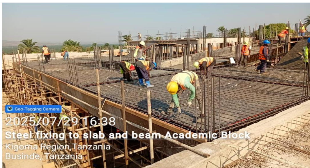
Plate 1: Steel fixing to slab and beam in the Academic Block.
