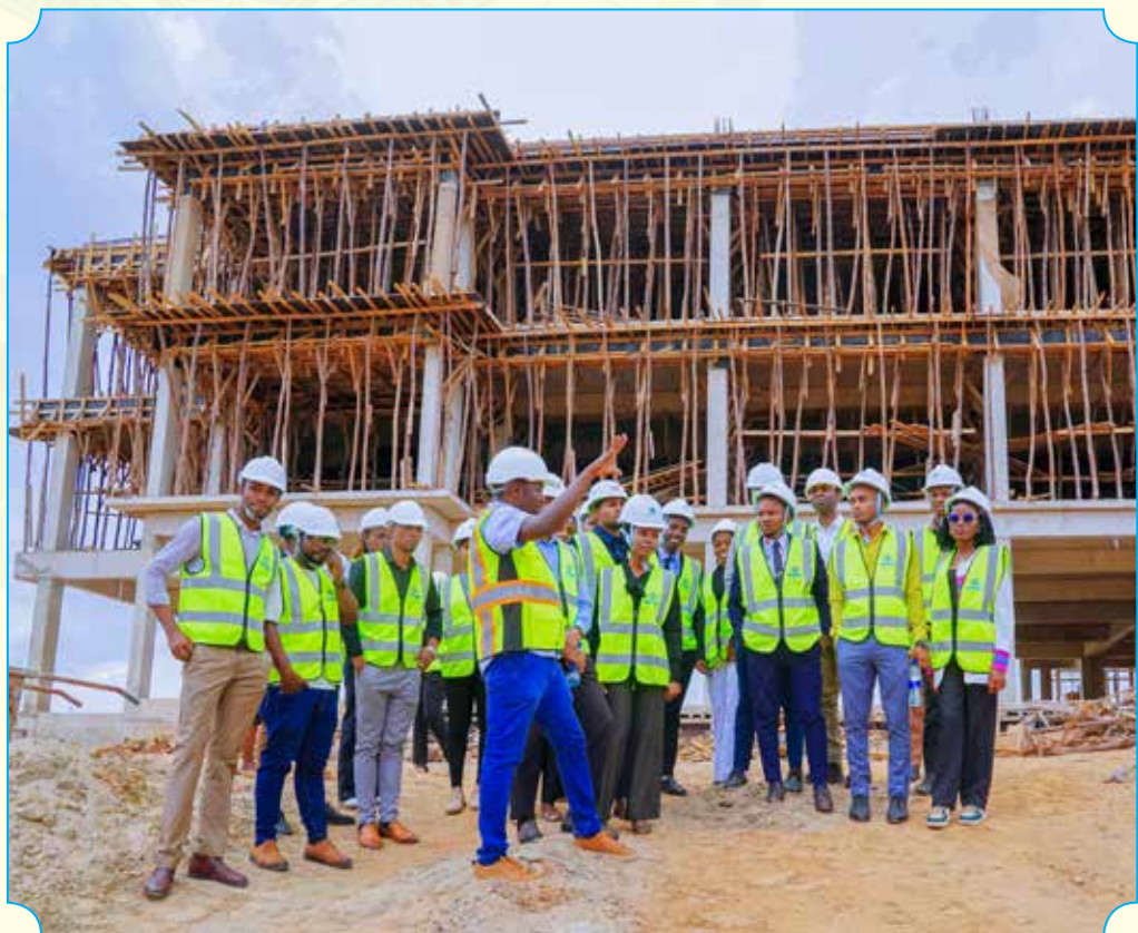
Engineer Shandrack Magoro giving a briefing on the progress of the ongoing construction works to MUHASSO leaders during their visit to Mloganzila Campus.
