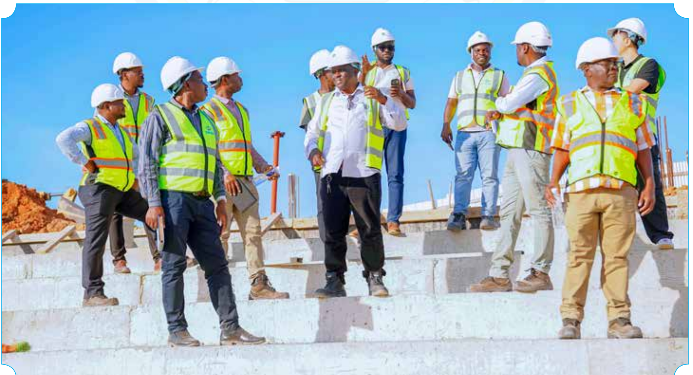
A team of experts from the Ministry of Education, Science and Technology inspecting the progress of the construction of the College of Medicine at Mloganzila Campus.
