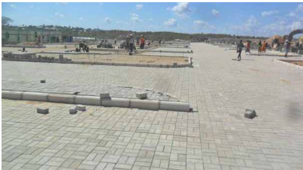
Installing cabstone for road, car park and paved area at North of the MUHAS Academic Medical Centre
