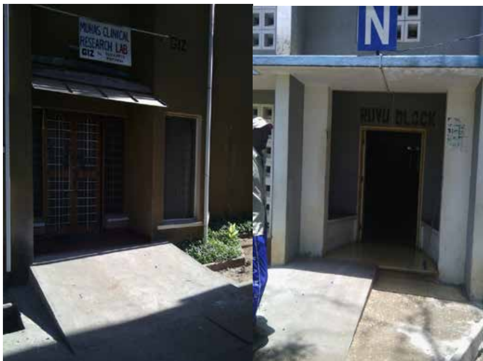
Ramps construction at at Offices and Hostel Buildings entrances
