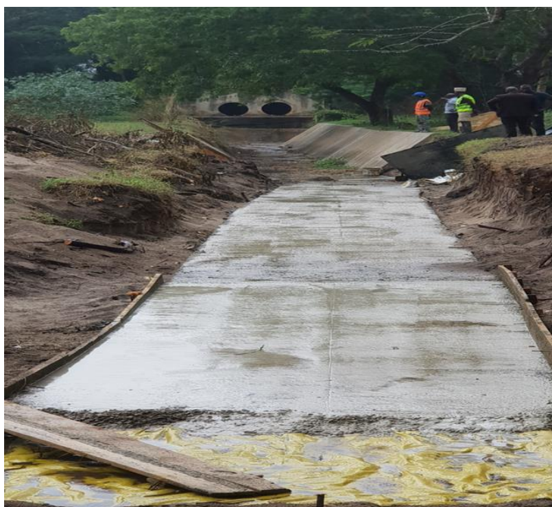
Figure 26: Construction of Stormwater Channel at Badeco Beach Plot Bagamoyo
