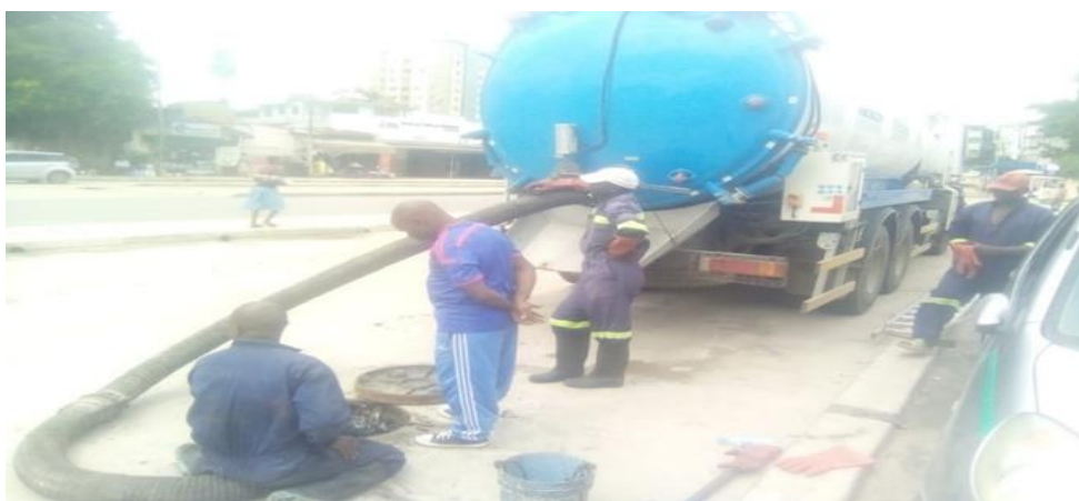
Figure 31: Executing Preventive Maintenance of the Sewer System at MUHAS main Campus
