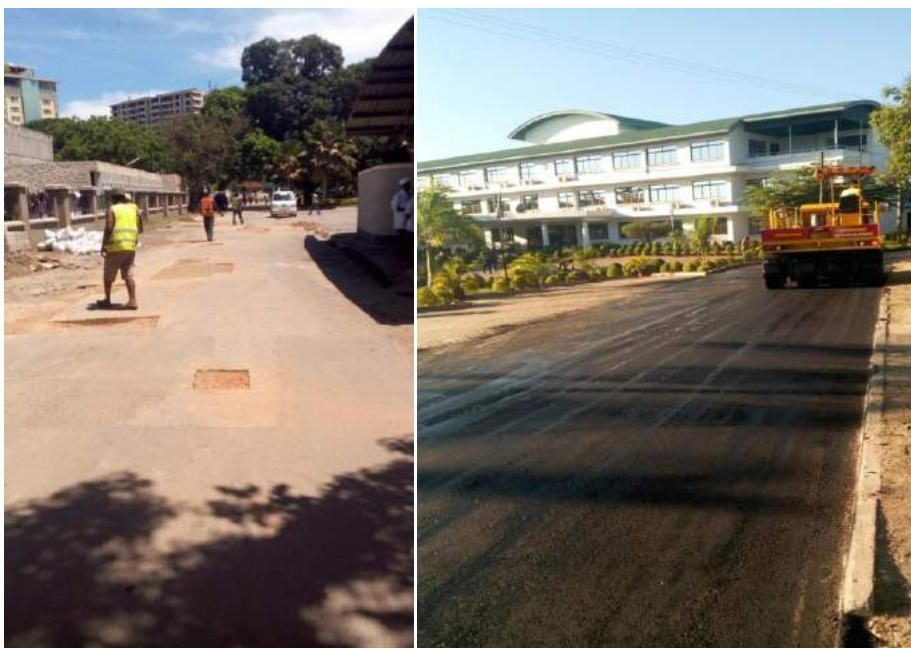
Figure 28: Cutting of Pot Halls and Tarmac laying at the Stretch of Road from MTC gate to HD CHPE building.
