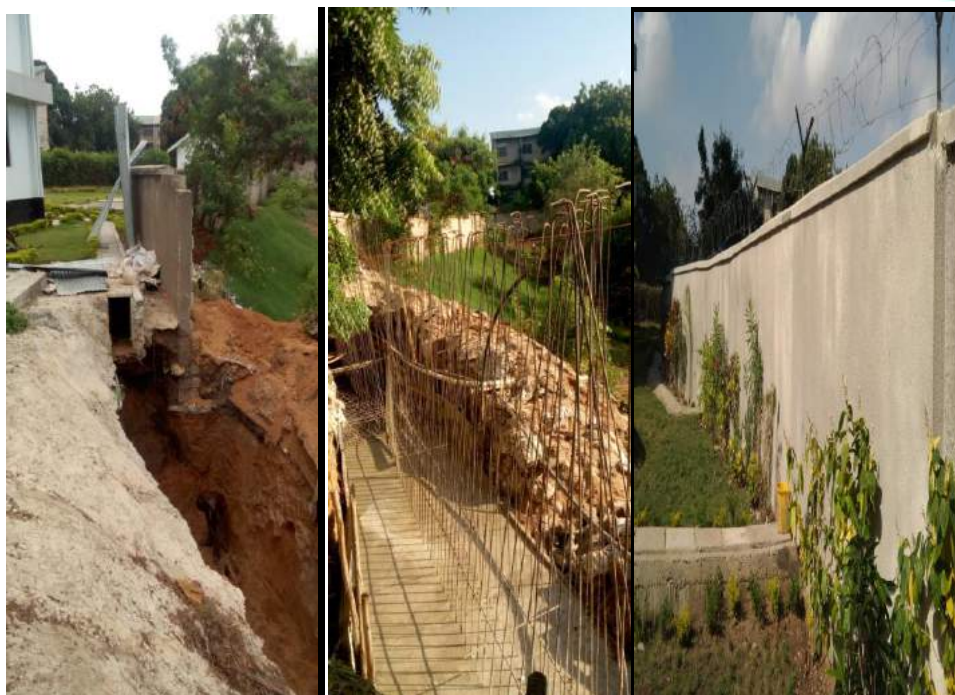
Figure 26: Wall Renovation at excavation stage, rebar setting and the final completed wall stage
